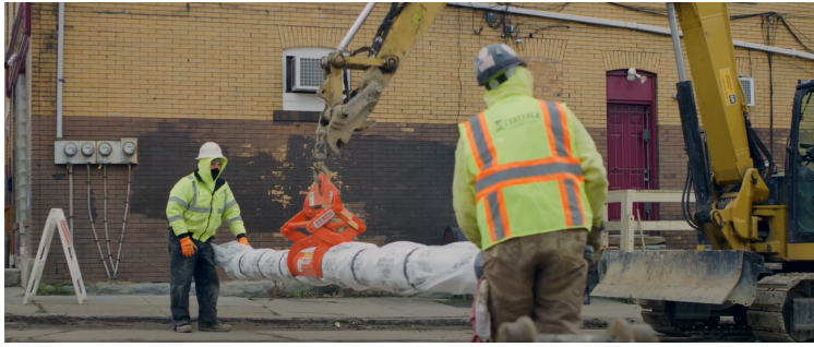
PWSA contractor crews installing a new water main.
