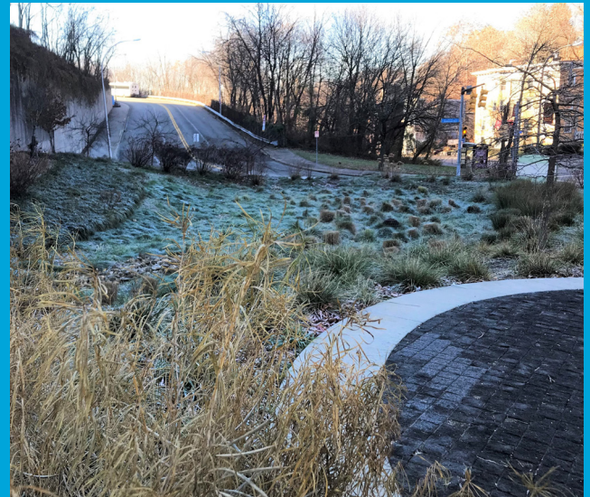
Our Centre and Herron stormwater project in the Hill District with a hint of frost in December 2021.
