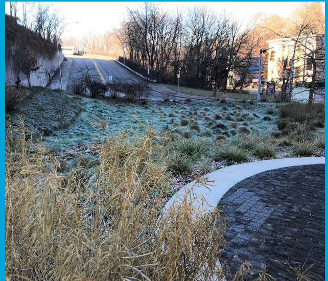
Our Centre and Herron stormwater project in the Hill District with a hint of frost in December 2021.
