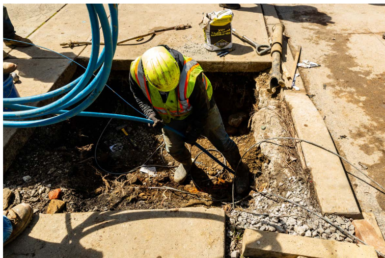
Funding received from PennVEST since 2018 has supported the removal of thousands of lead service lines from our drinking water system.
