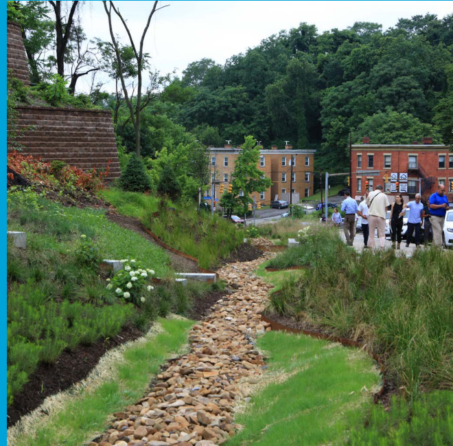
This cascading bioswale at Centre and Herron in the Hill District is 585 feet long!
