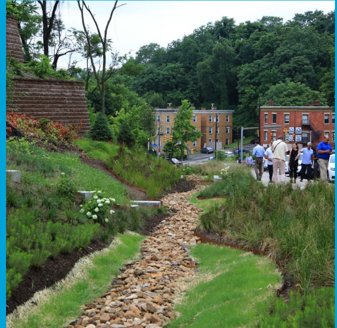
This cascading bioswale at Centre and Herron in the Hill District is 585 feet long!
