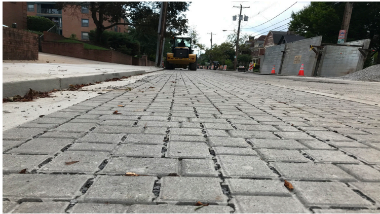
Permeable pavers installed at Kentucky Ave. in Shadyside
