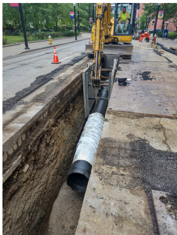
Crews install new water main on Forbes Avenue in The Bluff
